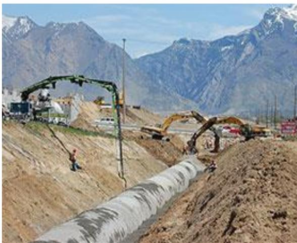
**Picture 1:** Piping of the Provo Reservoir Canal in Utah, Source: Bureau of Reclamation, Upper Colorado Region
